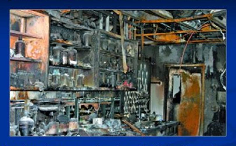
Grad students were loading 10-12 bottles of hexane onto lab shelves when a shelf collapsed. Over 40 gallons of hexane were present in the lab.
